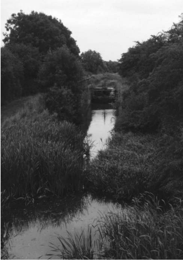
A lock on the Grantham Canal awaiting restoration
