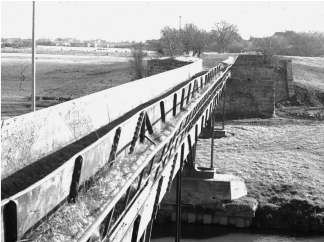
The cast iron aqueduct at Longdon-on-Tern, Telford's prototype for the aqueduct at Pontcysyllte.
