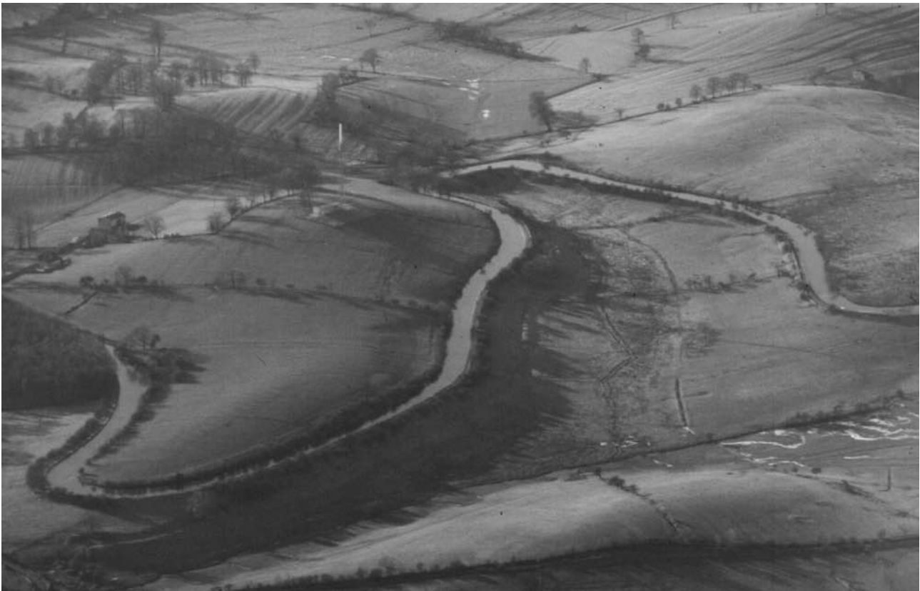
A typical English contour canal, the Leeds & Liverpool Canal in the Pennine hills.
