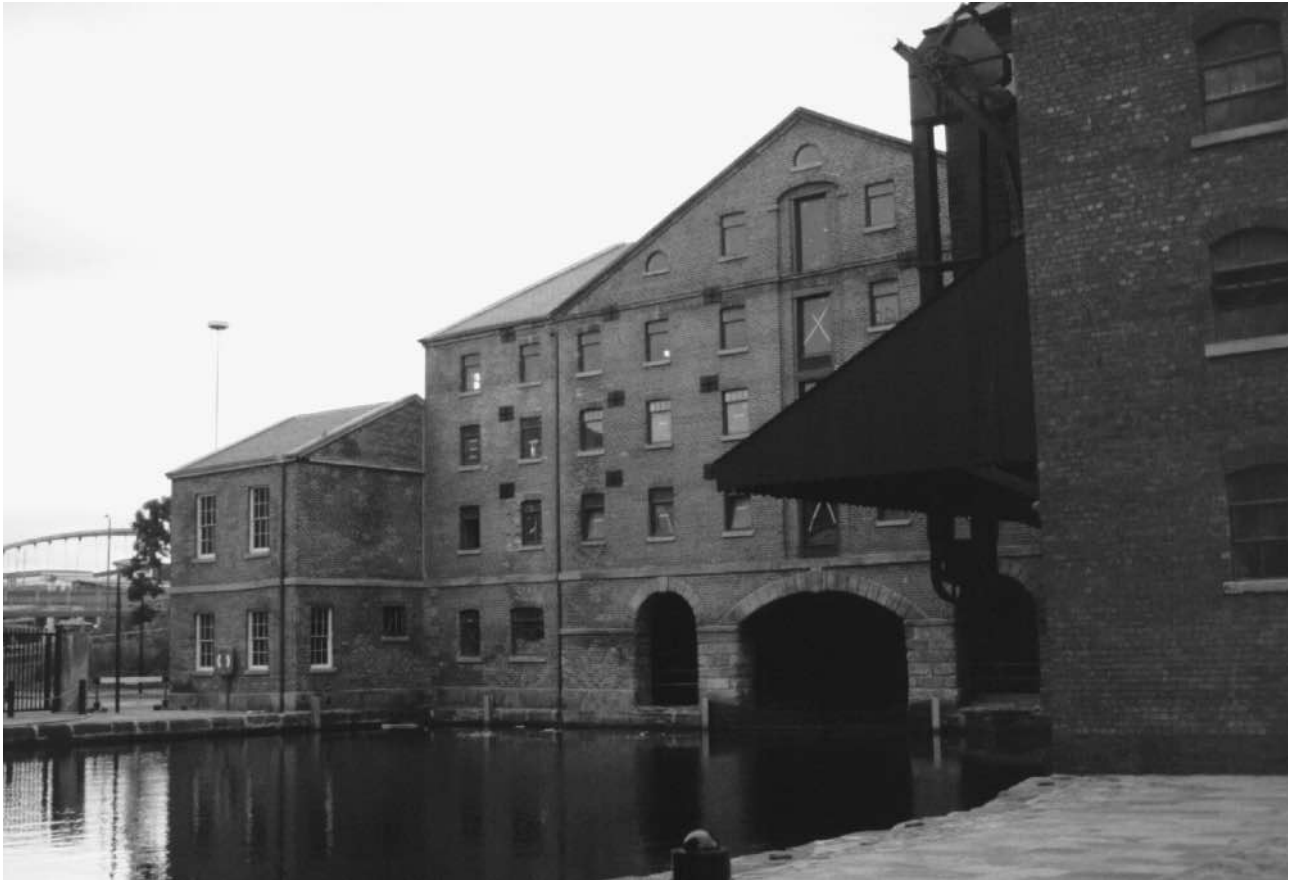
The older of the two recently restored Sheffield warehouses which has been converted into offices.
